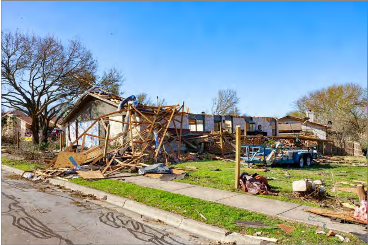
Figure 14-3. Tornado-Damaged Home in City of Round Rock, March 21, 2022 7
