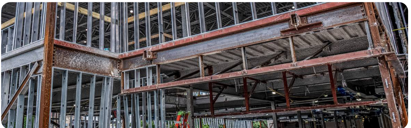
Construction on the Griffith Building Remodel
