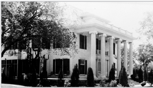
The Nelson-Crier House, built 1895-1900, remodeled 1931, is a Round Rock historic landmark and a Recorded Texas Historic Landmark (RTHL).
