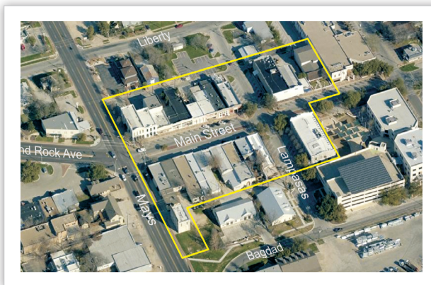
The Commercial Historic District encompasses 25 properties within four city blocks.
