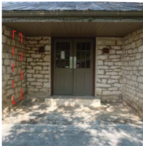
Original door opening with modern doors at east elevation; Dotted red outline of possible historic door at left
