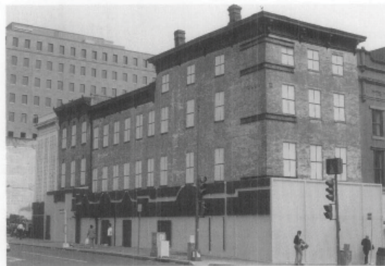
Figure 11. Urban buildings often need additional protection from unwanted entry and graffiti. This commercial building uses painted plywood panels to cover expansive glass storefronts and chain link fencing is applied on top of the panels. The upper windows on the street sides have been covered and painted to resemble 19th century sash. Photo: Thomas Jester, NPS.
