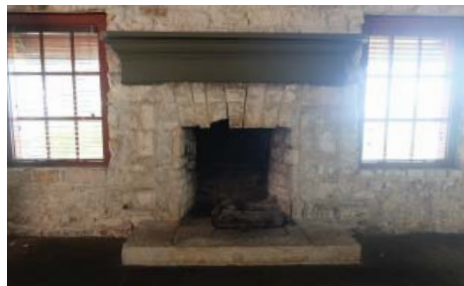
North fireplace with painted mantel and chipped masonry
