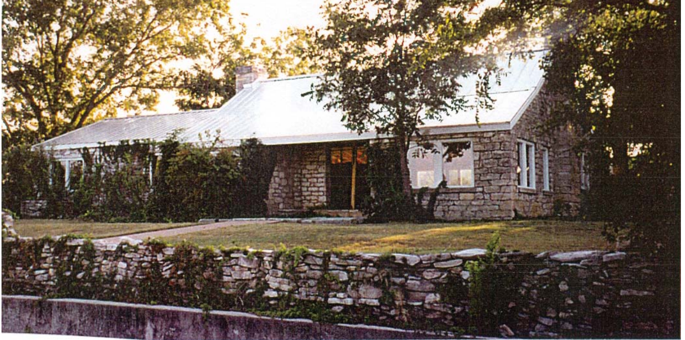
Figure 11. 1994 Renovation: South addition, new metal roof, replacement windows, new landscaping and entryway steps (Source: City of Round Rock)
