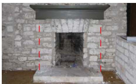
South fireplace with red lines indicating the outline of an early mantel
