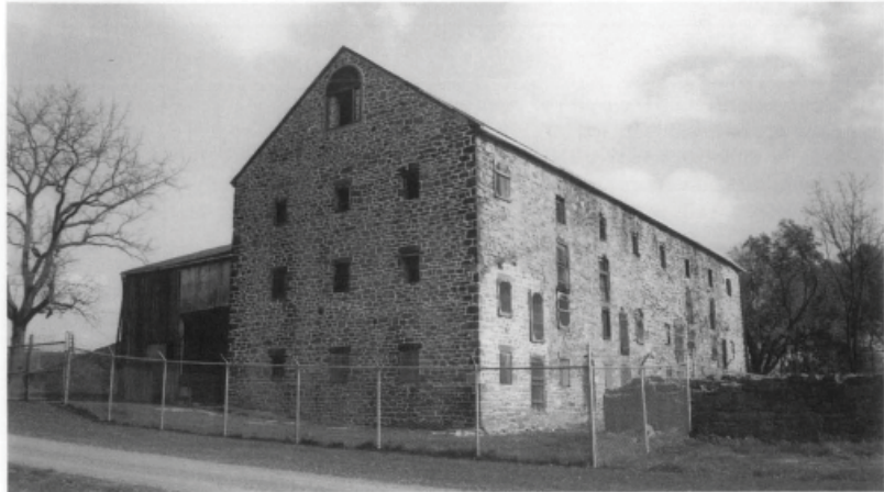
Figure 24. Once mothballed, a property must still be monitored and maintained. The openings in this historic barn have been modified with a combination of wood louvers and metal mesh panels which require little maintenance. The grounds are regularly mowed, even inside the chain link security fence. Photo: Williamsport Preservation Training Center, NPS.
