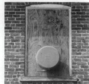
c. The exhaust fan has tamper-proof housing.
