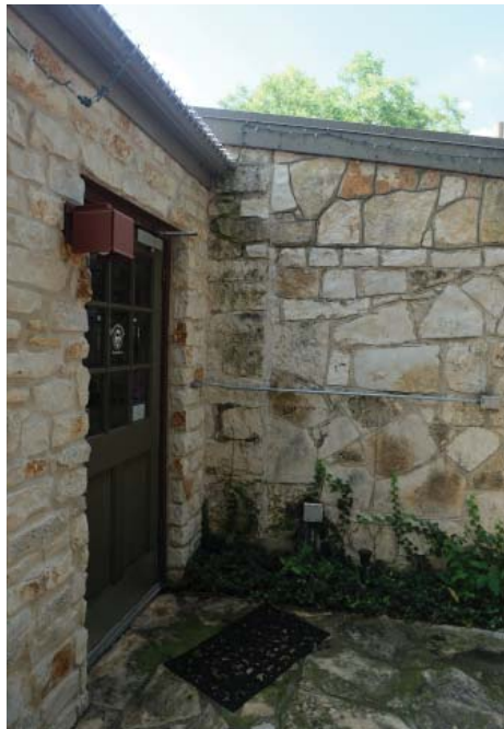
Change in stone from historic building (left) to new addition (right) at north side
