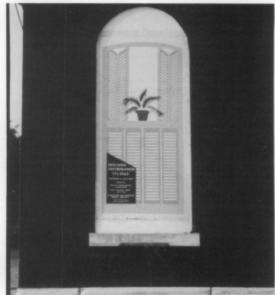
Figure 15. Painting trompe l'oeil scenes on plywood panels is a neighborhood friendly device. In addition, the small sign at the bottom left corner gives information for contacting the organization responsible for the care of the mothballed building. Photo: Lee H. Nelson, FAIA.
